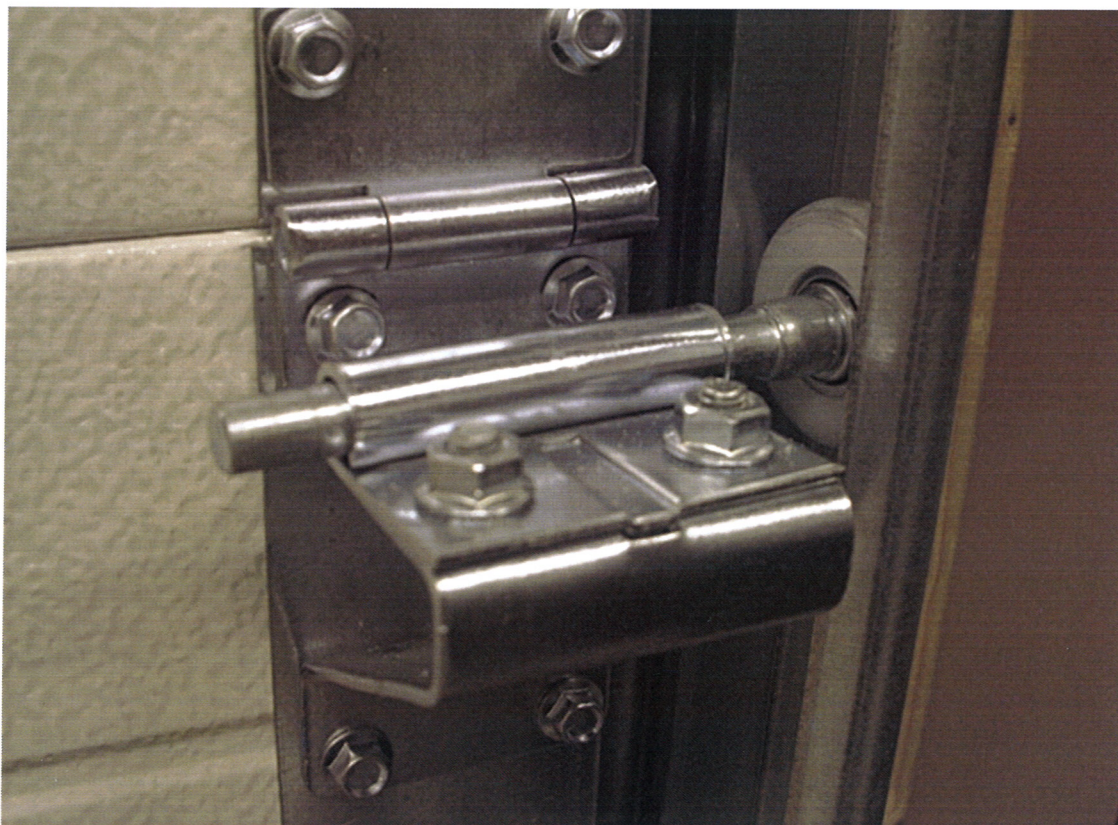
Figure 3. Side hinge, slide and roller.
