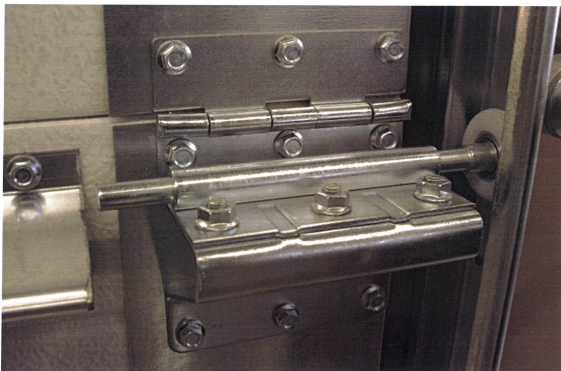
Figure 3. Side hinge, slide and roller.
